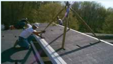
Panels set into place
