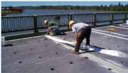
Splice strips installed over field joints
