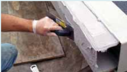
Adhesive applied at field joint
